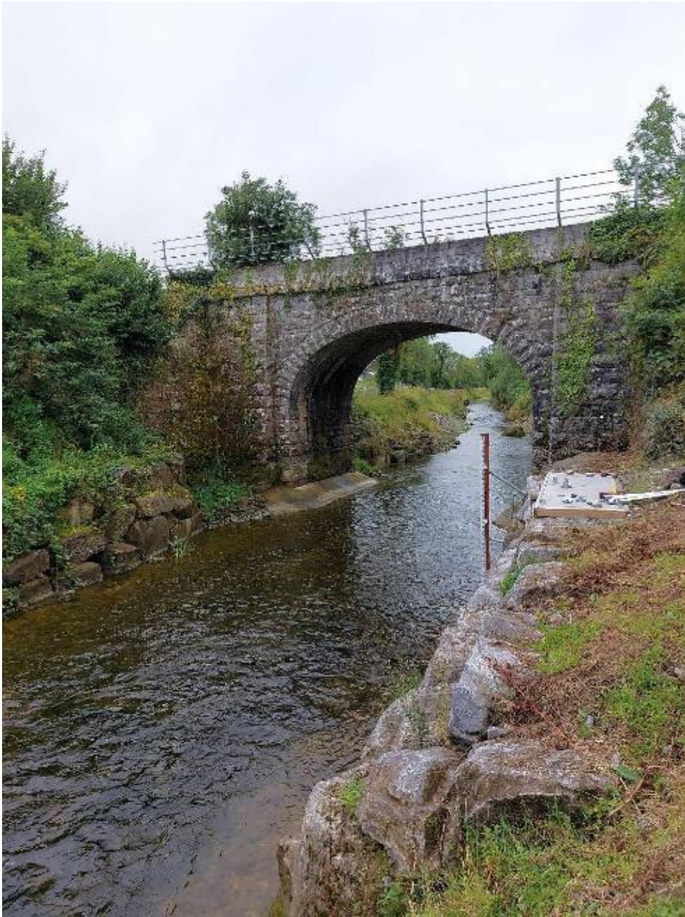
Figure 1 New OPW Hydrometric Station Craughwell 29007 (looking west).
