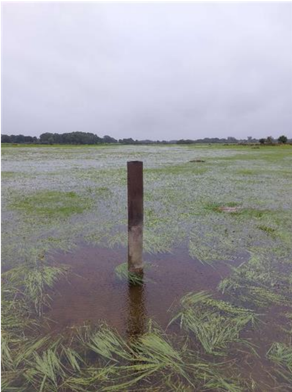
Figure 12 ID 9 – Monitoring well (condition unknown)
