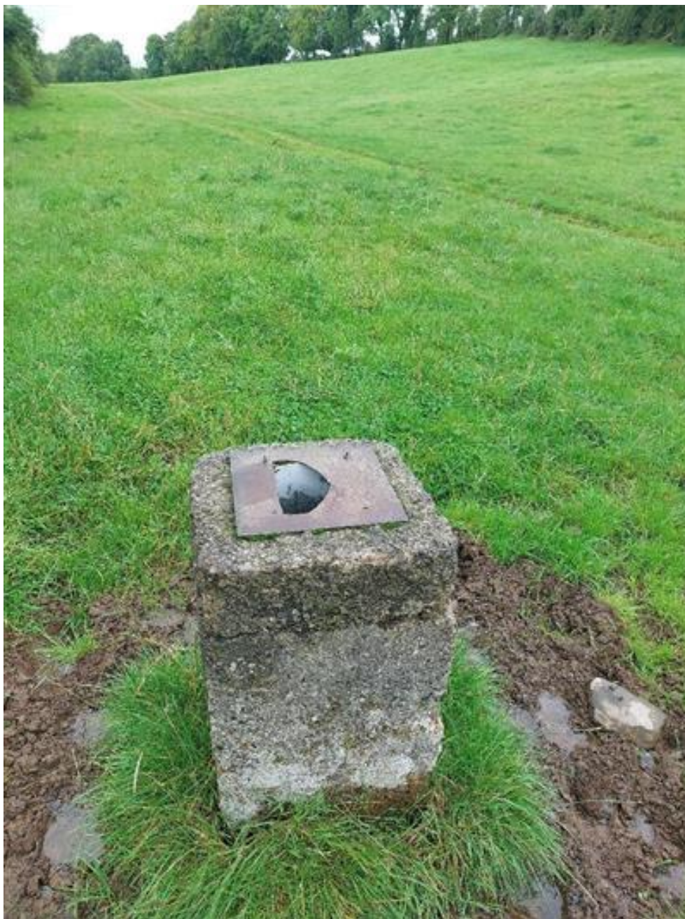
Figure 13 ID 10 – Monitoring well (condition unknown)
