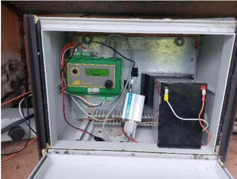
Figure 3 Data logger at the Aggard Bridge 29010 Hydrometric Station.
